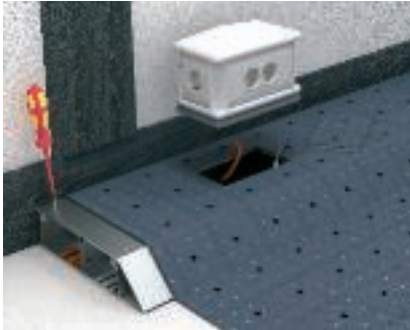
Floor covering work, mounting lid For lids with installation or setup openings, the protective mounting lids are removed and, after application of the floor covering, the mounting openings are cut out cleanly.
