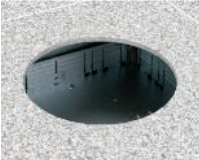
Laying the floor covering Lay the floor covering up to the mounting opening for GRAF9.
