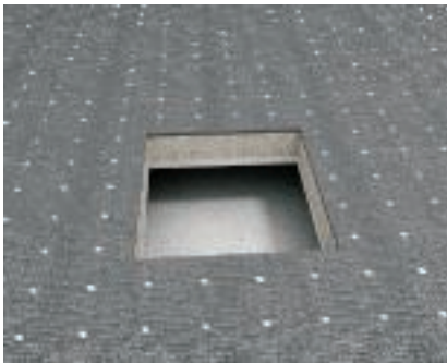
Use of square screed protection cover Square lined bodies create an installation opening for height-adjustable square cassettes. Note: Not suitable for service outlets.
