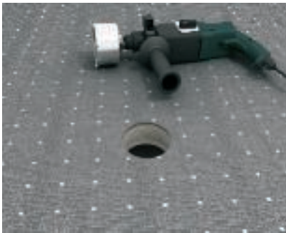
Creation of an installation opening by drilling Create an installation opening with a crown drill.
